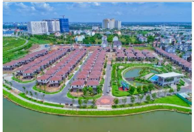
Figure 8: Kikyo Valora Project
