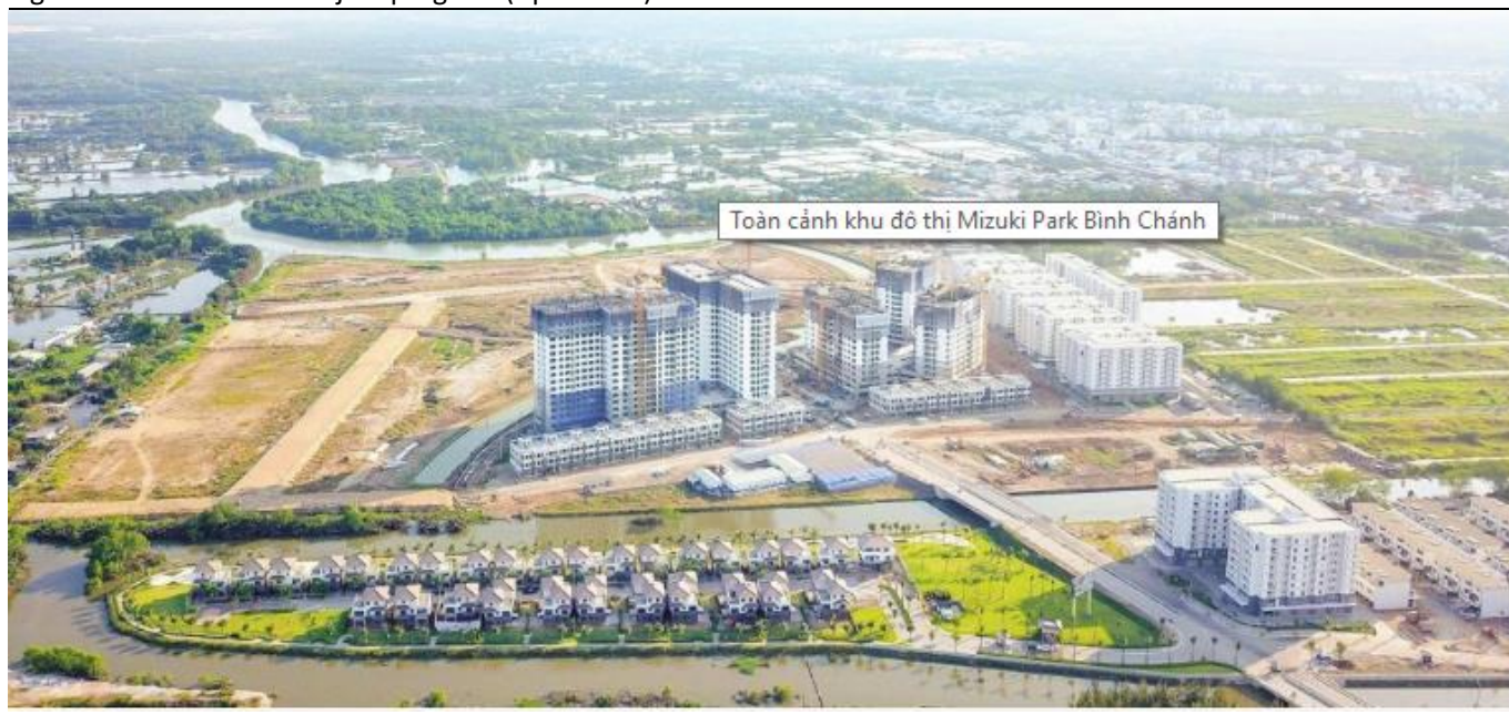
Figure 23: Mizuki Park Project progress (April 2019)
