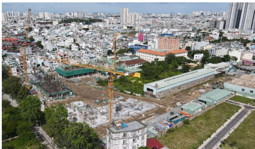
Fig 5. KDH – Construction progress of Privia project
