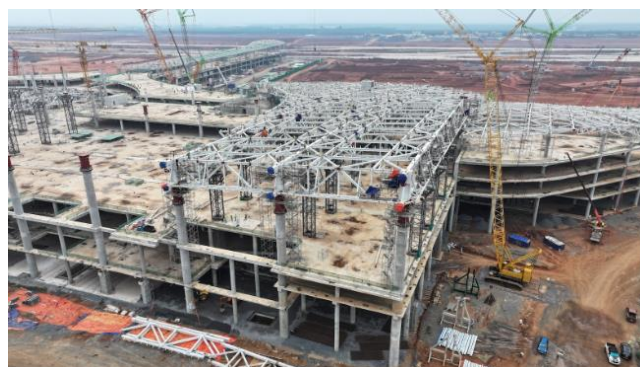
Fig 3. ACV - Long Thanh International Airport progress
