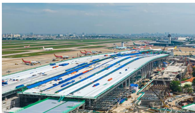
Fig 2. ACV - Tan Son Nhat T3 Passenger Terminal progress
