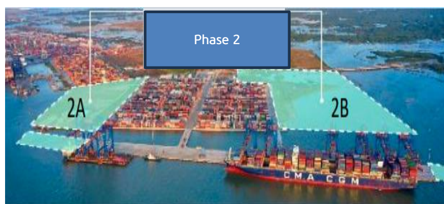
Fig 8. GMD – Gemalink's construction progress
